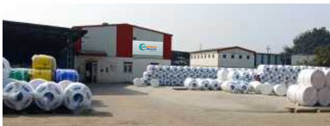
Manufacturing Plant - Sikandrabad (U.P.)
